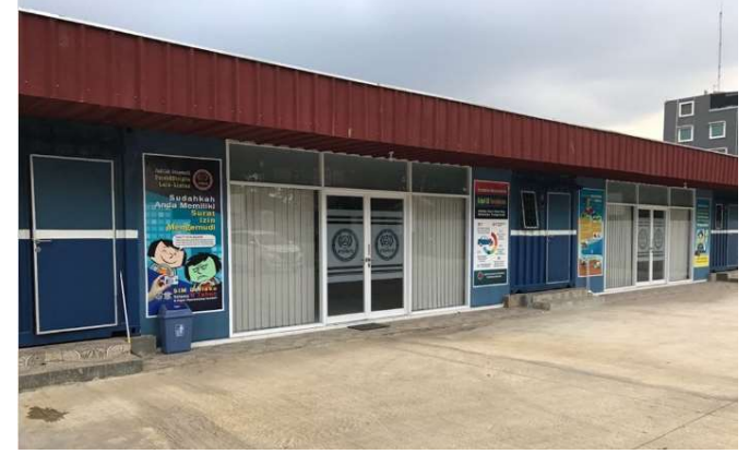
Kantor Operasional LSP-TGI
